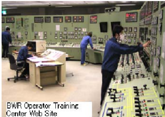
Picture-1: 1st generation control panel
