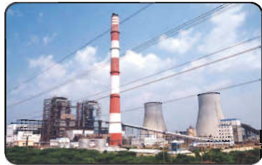
Thermal Power Station-Neyveli
