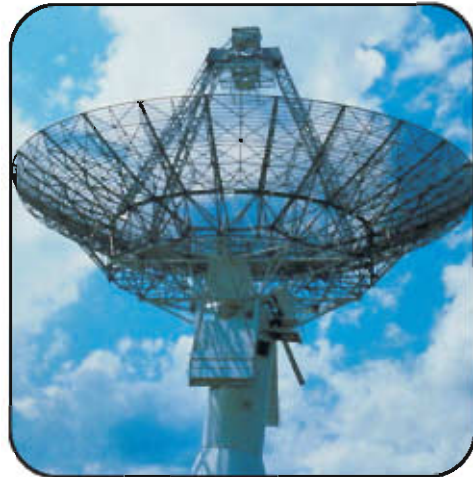
Tele Communication Antenna
